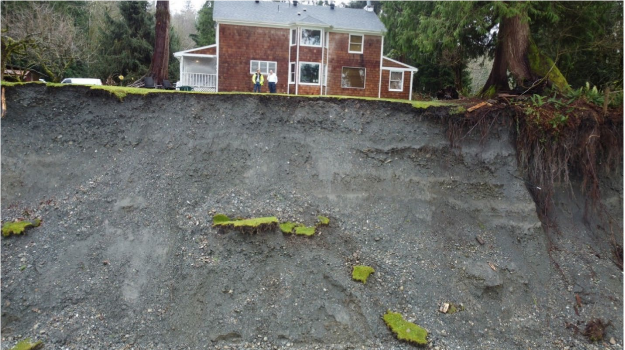
Figure 16: Residential structure adjacent to active slope failure along South Skagit Highway, where flooding and slope instability resulted in evacuation orders and unsafe-to-occupy conditions. This home is located between Hamilton and Sedro-Woolley, Skagit County, WA.
