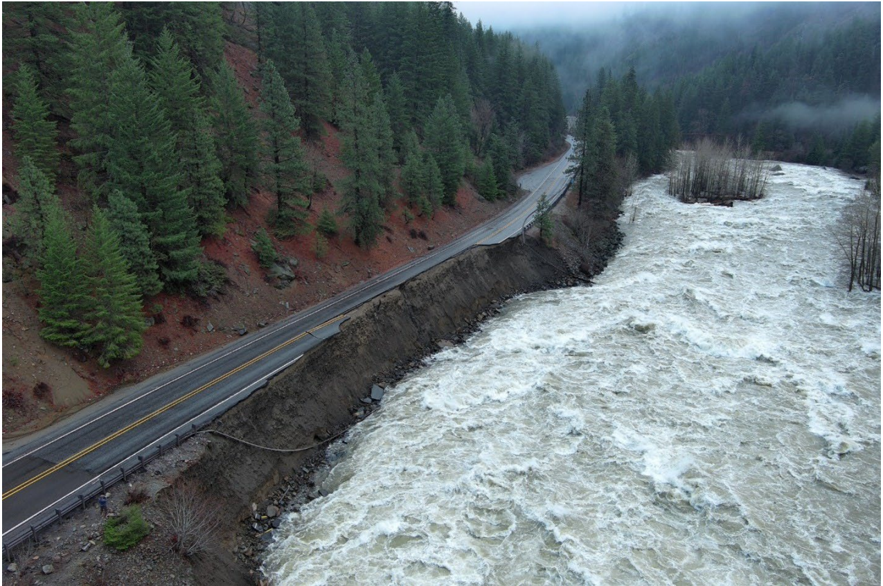
Figure 34: Large washout from December 12, 2025, of US 2, west of Leavenworth, Chelan County, WA.
