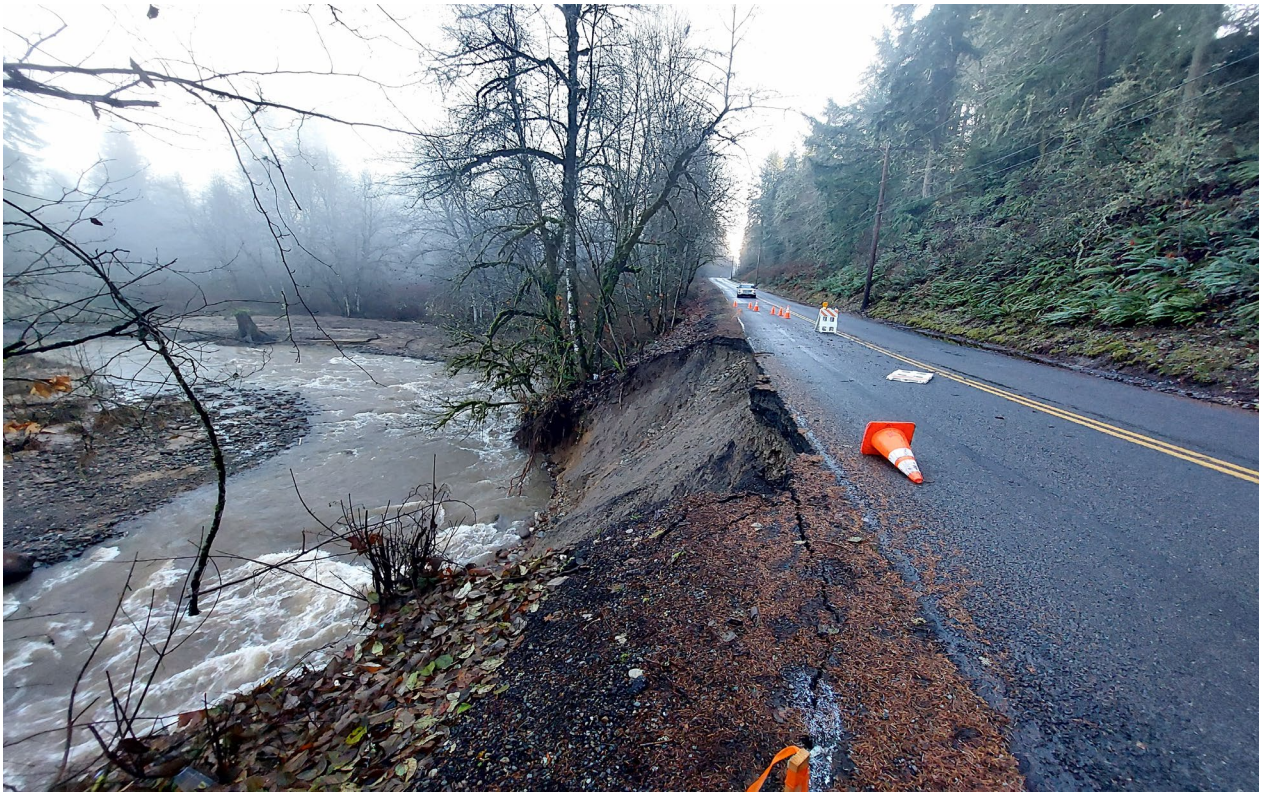
Figure 33: Wilkeson Creek flooding causing landslide impacting Johns Road E., Pierce County, WA.
