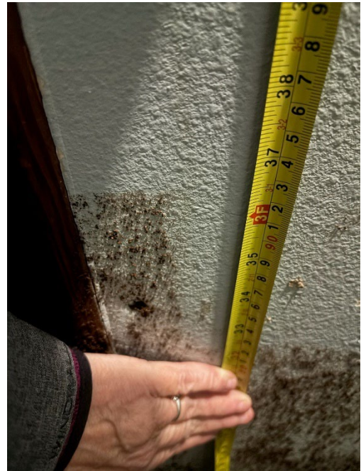
Figure 15: Mold growing on walls in residence.
