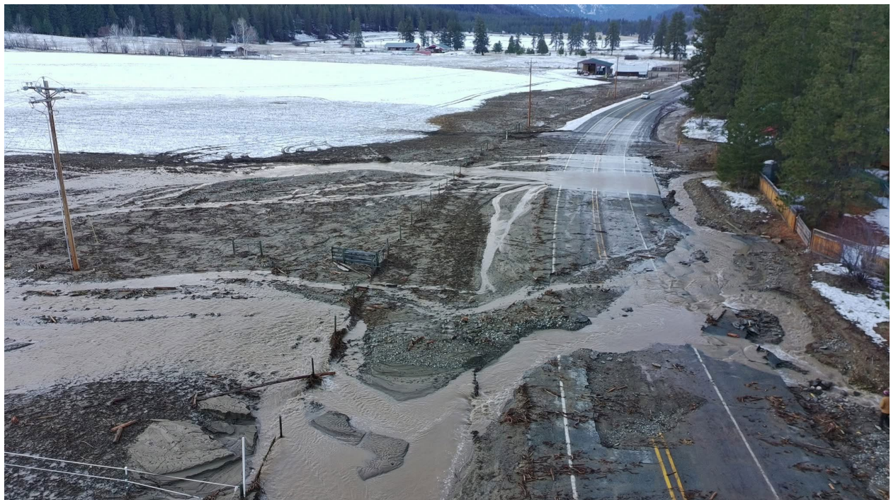
Figure 45: Roadway washout on U.S. Highway 20 Skagit County, WA.
