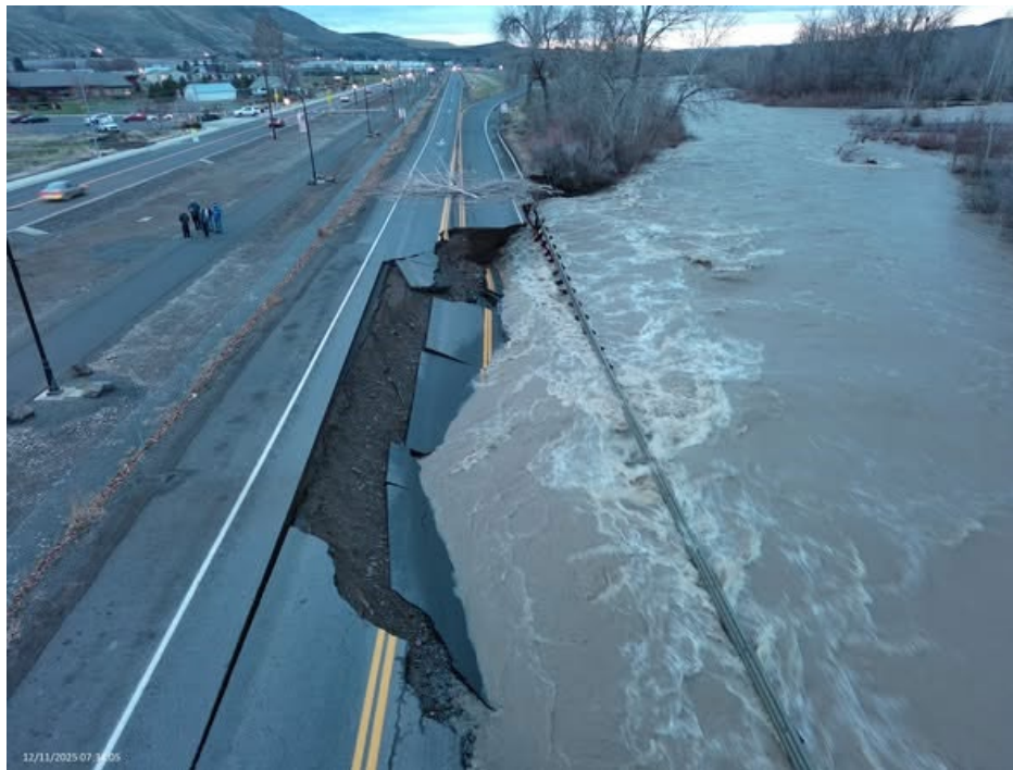
Figure 40: A section of US Highway 12 destroyed in Naches, Yakima County, WA.
